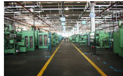
1. Feeders continued with load.
